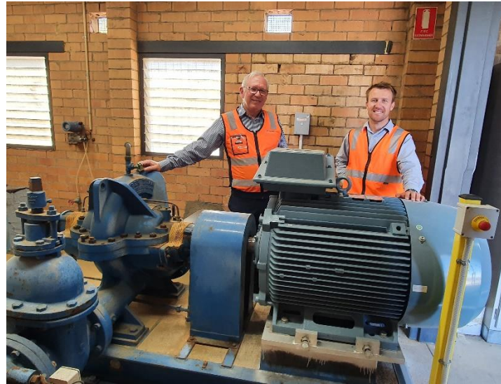
(L-R): Anthony Merrett from Remtron and Mitchell Palmer from AlburyCity Council, beside ABB's M2BAX IE3 high efficiency motor.
